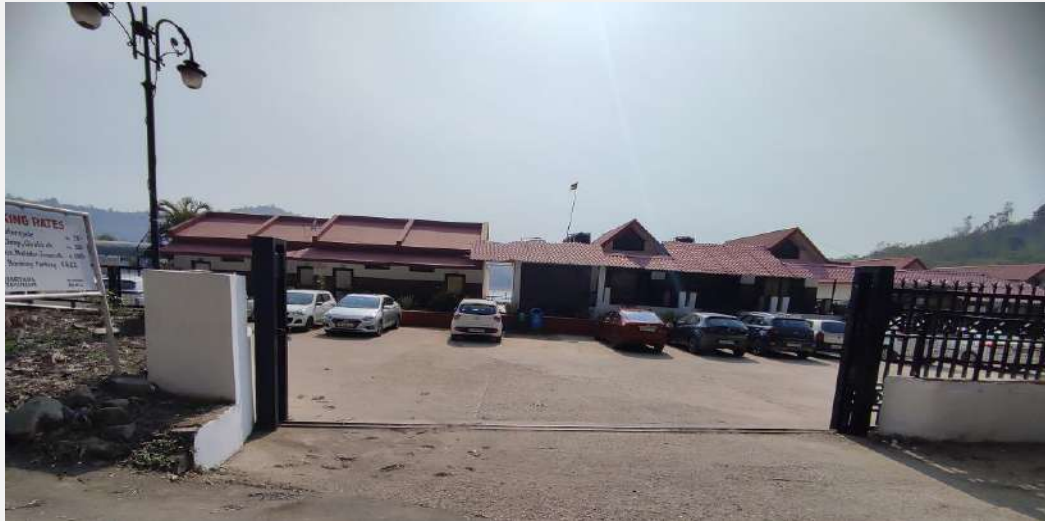
Figure 6-6 Entrance area lacks any registration/holding area
