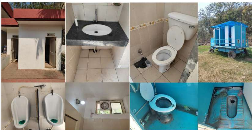
Figure 6-10 Condition of existing toilet block
